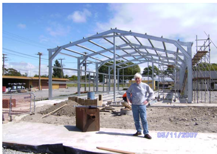
Phil Mitchell and the additional new facility taking shape
